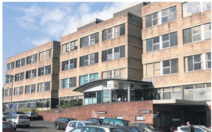
RSH - Department of Psychiatry building (not in use)
